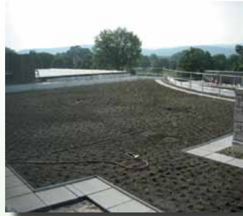
Initial Green Roof Planting
